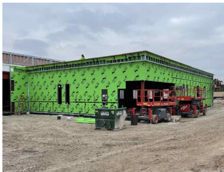
District office exterior wall sheathing is nearly complete.
