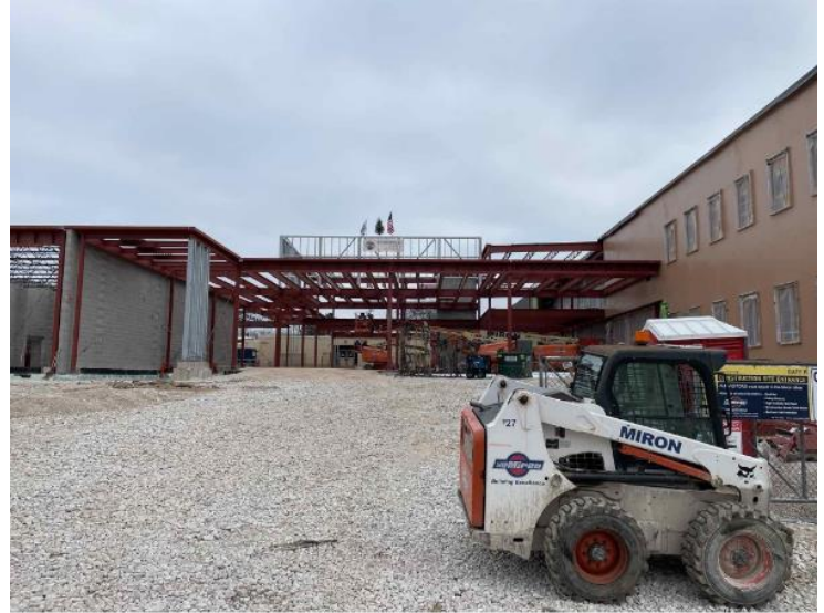
All building mass structural steel framing is complete!
