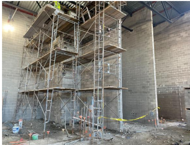
Masonry stage walls in gym.
