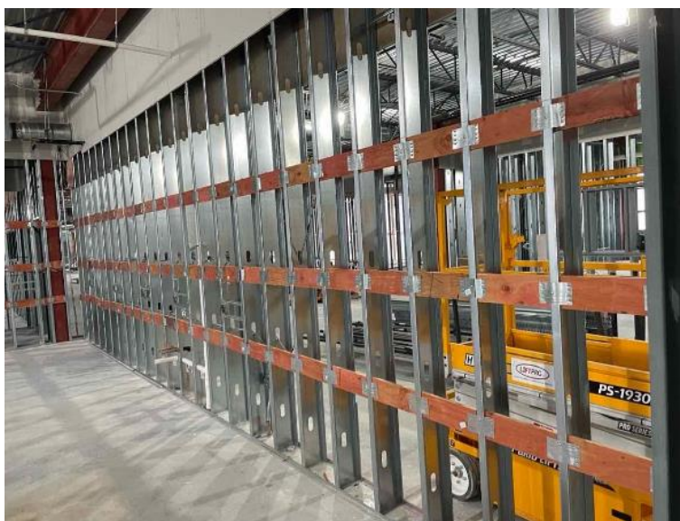
Completed in-wall blocking for supporting new cabinetry in classrooms.
