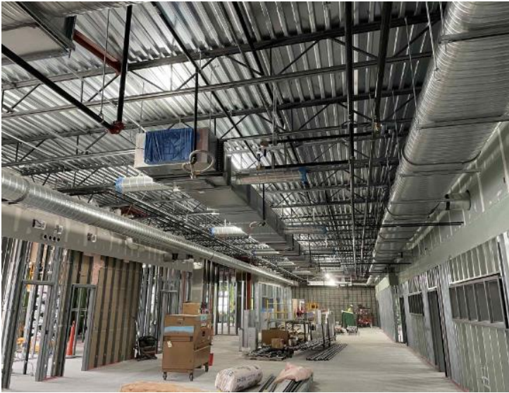
Mechanical ductwork installed in the classroom wing, second floor.
